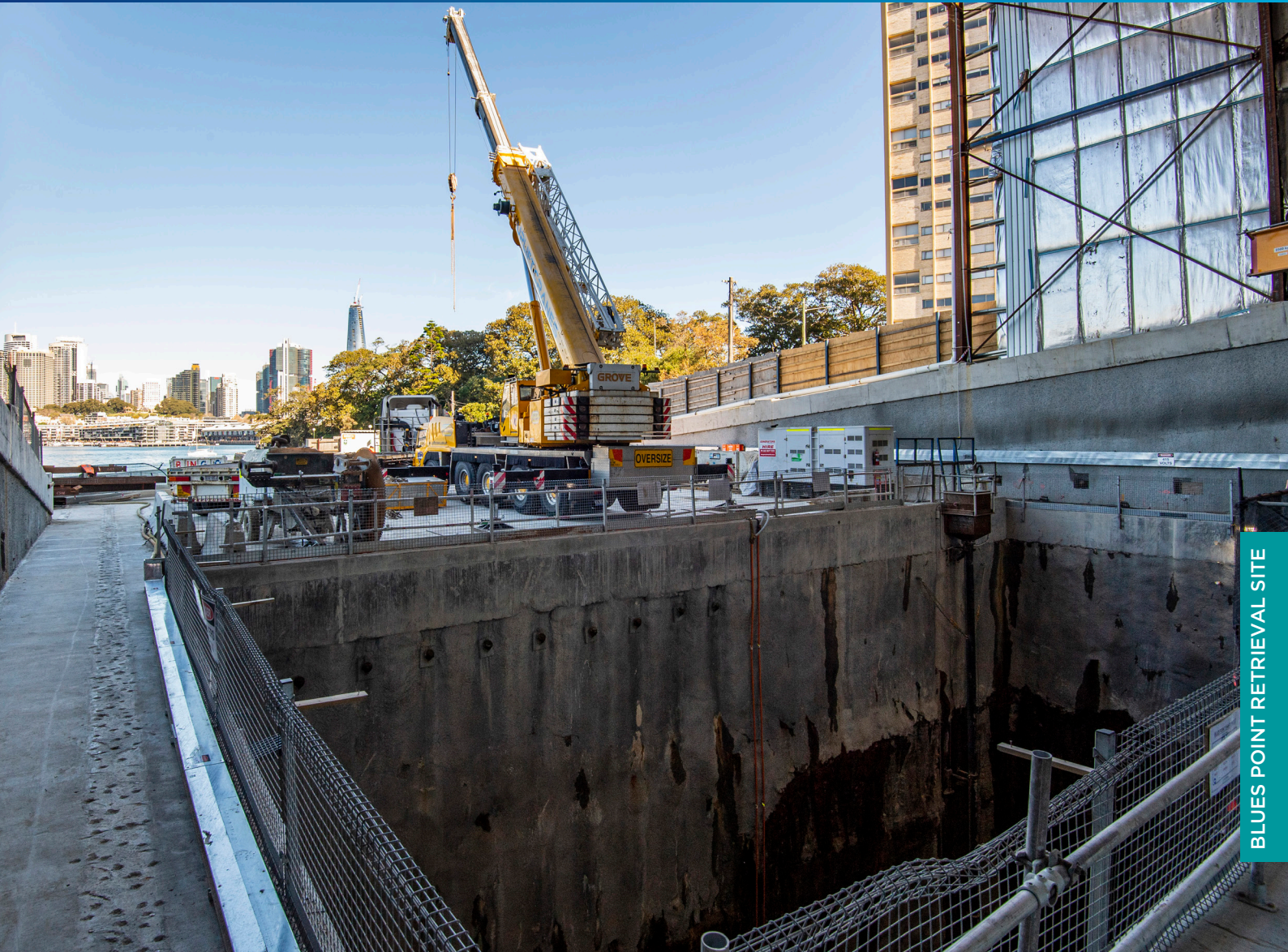
The top of the Blues Point shaft where a portion of the acoustic shed has now been removed
