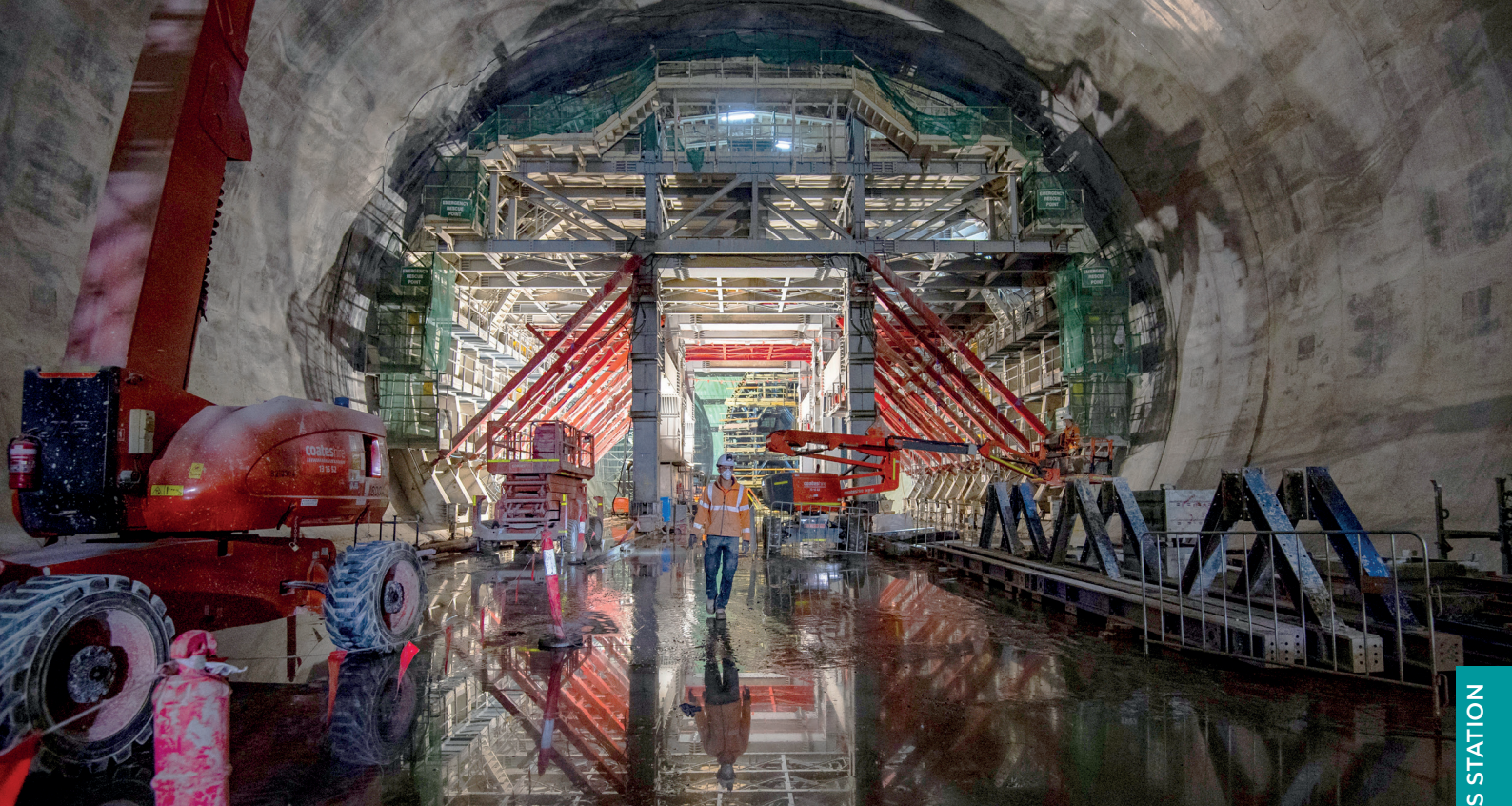
Formwork structures are an impressive sight inside of the Victoria Cross cavern
