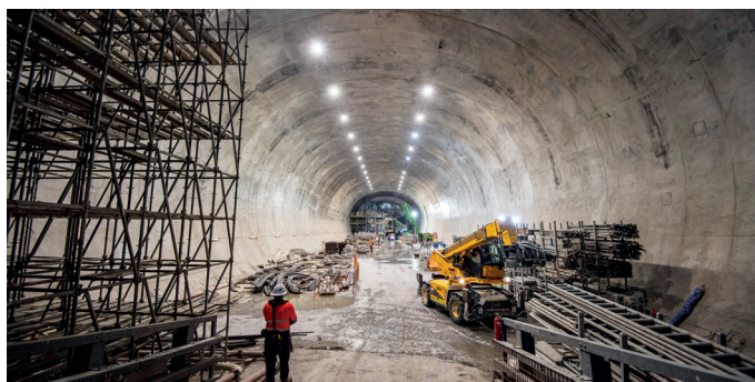
The Victoria Cross cavern is the largest rail cavern in Australia
