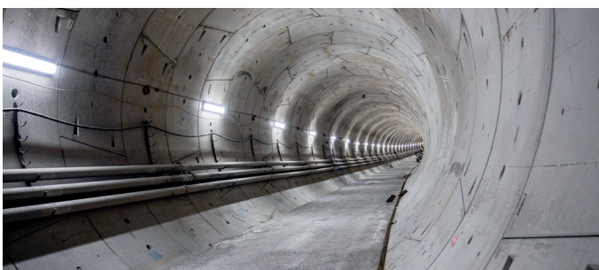
Sections of completed tunnels are now ready for track installation
