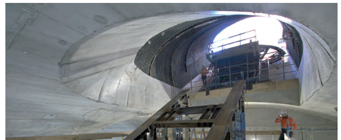
The location of the future escalator barrel at Martin Place Metro Station
