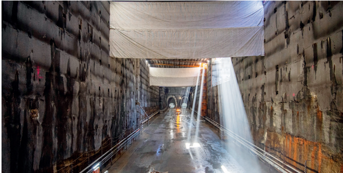
Inside the completed Crows Nest Station box
