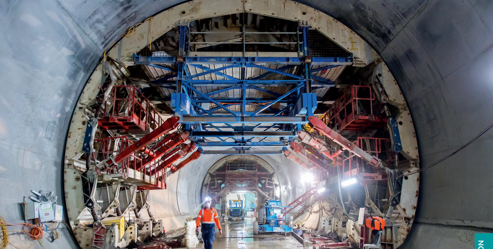
Movable formwork inside the cavern tunnels at Pitt Street Station
