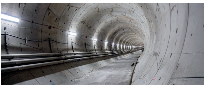
Sections of completed tunnels are now ready for rail track and systems installation
