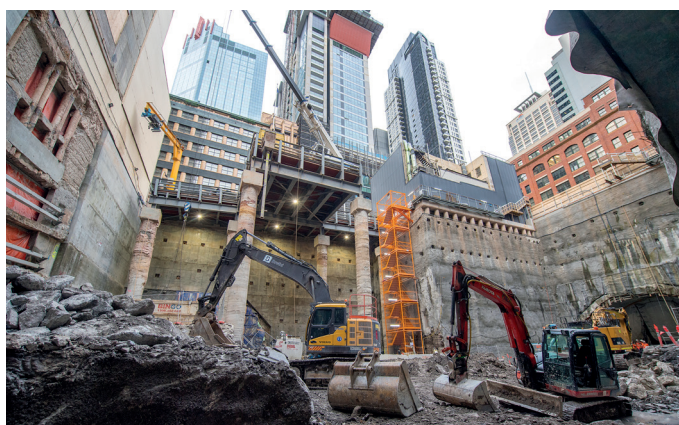
Pitt Street South shaft being excavated
