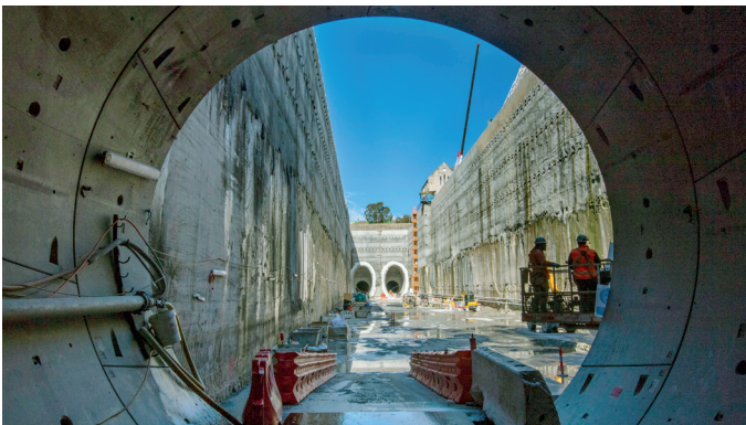
The Waterloo site has now been handed over to the integrated station development team
