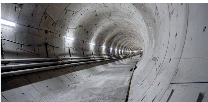
Sections of completed tunnels are now ready for rail track and systems installation
