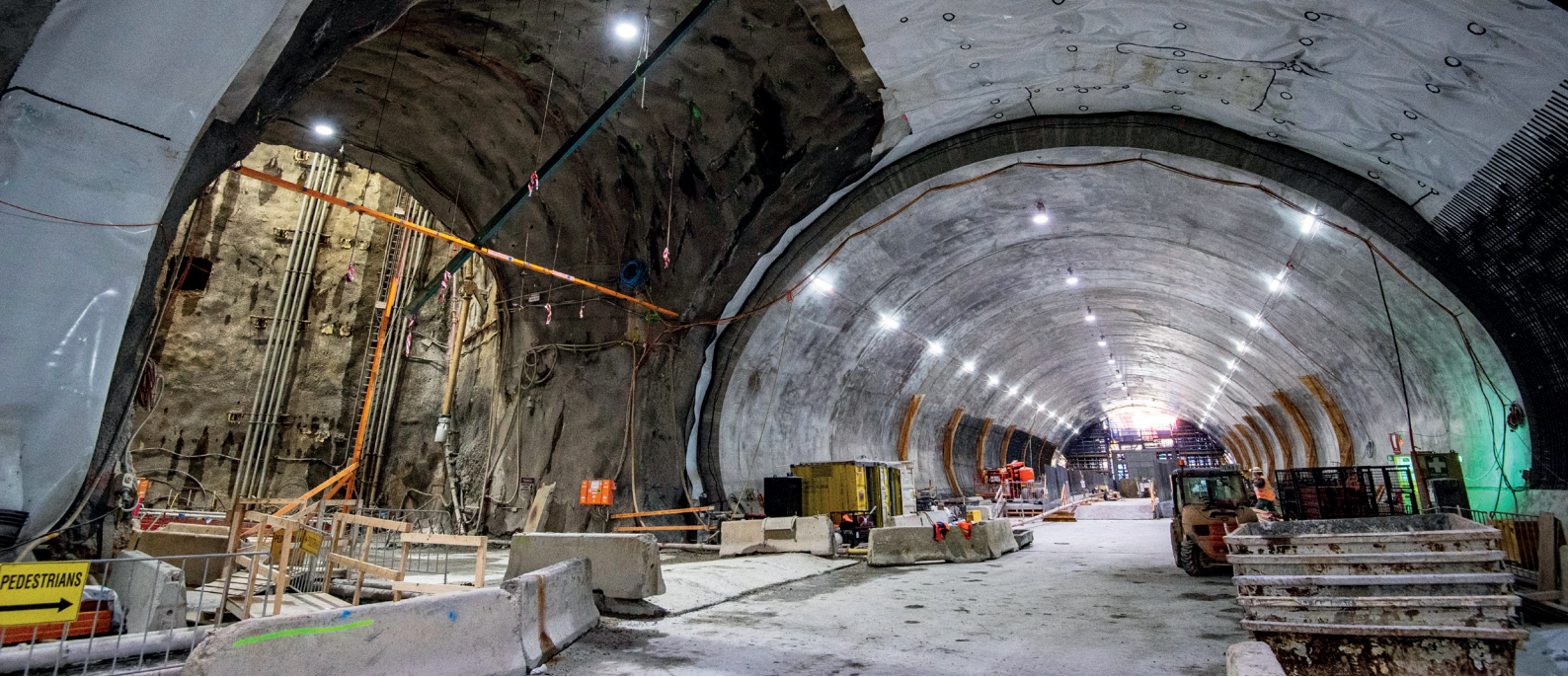
Concrete work inside the crossover cavern at Barangaroo
