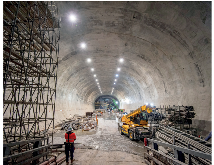
The Victoria Cross cavern is the largest rail cavern in Australia
