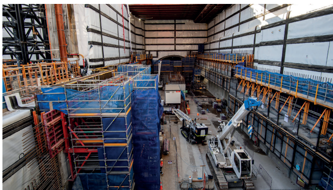
Perimeter wall construction inside the Barangaroo Station box
