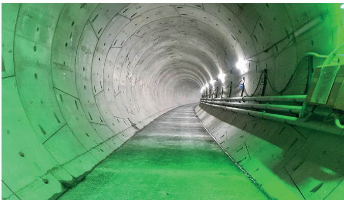
A look inside a the tunnel with the base slab complete
