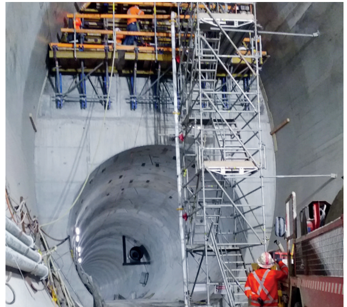
Headwall construction at Crows Nest station
