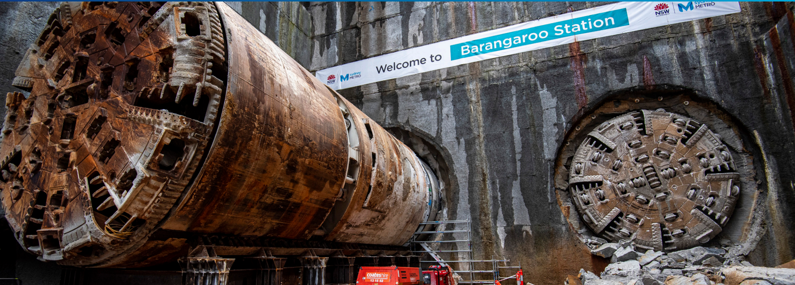
TBM Mum Shirl arrives at Barangaroo to mark the completion of the southern section of tunnelling
