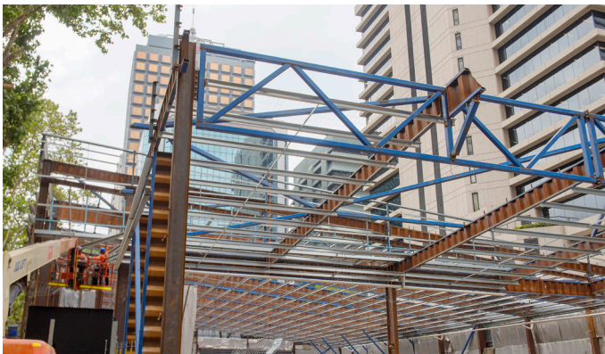
The acoustic shed at Victoria Cross is being demolished
