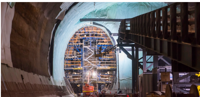
Formwork inside the cavern
