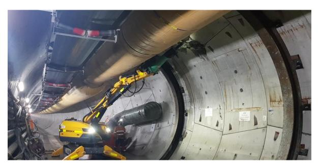
Cross passages are excavated using rock hammers like the one pictured above.
