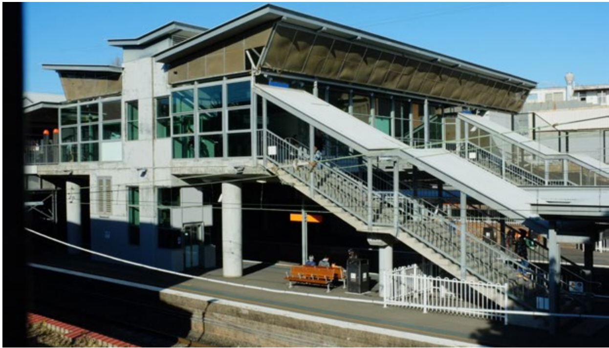
Figure 4.26 Existing stairs to platforms
