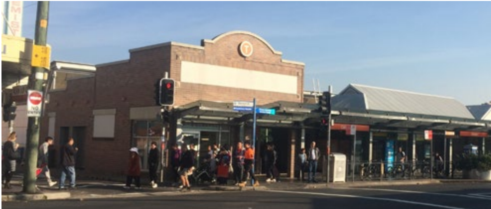
Figure 4.17 Existing 1990s corner building and parapet
