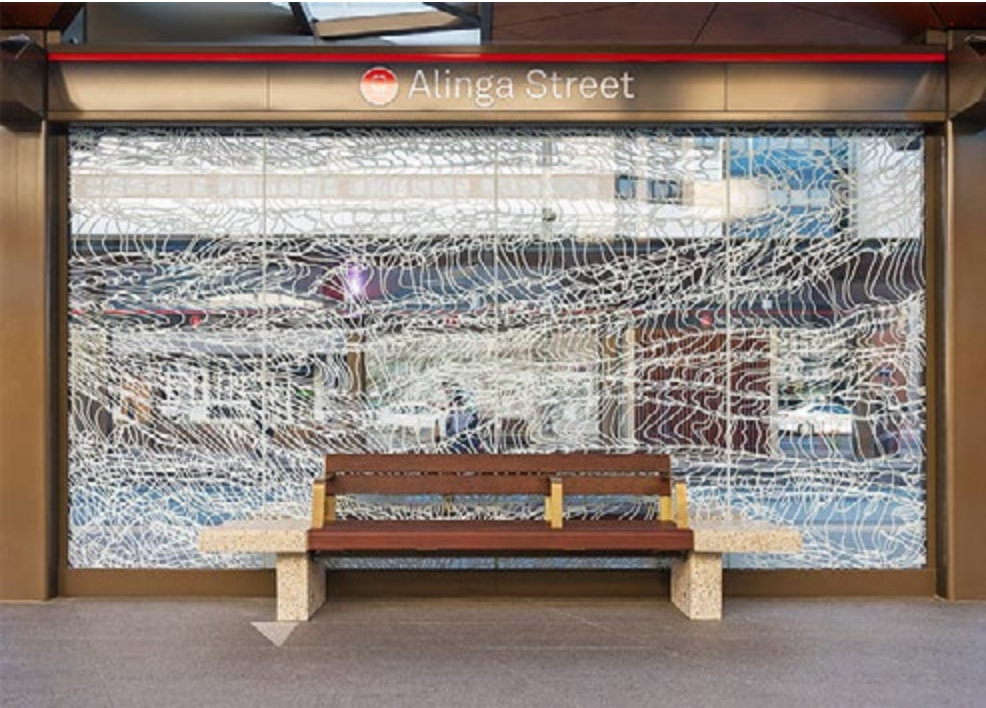
Figure 4.36 Example of glazed artwork screens at Canberra Lightrail. Art by Hannah Quinlivan
