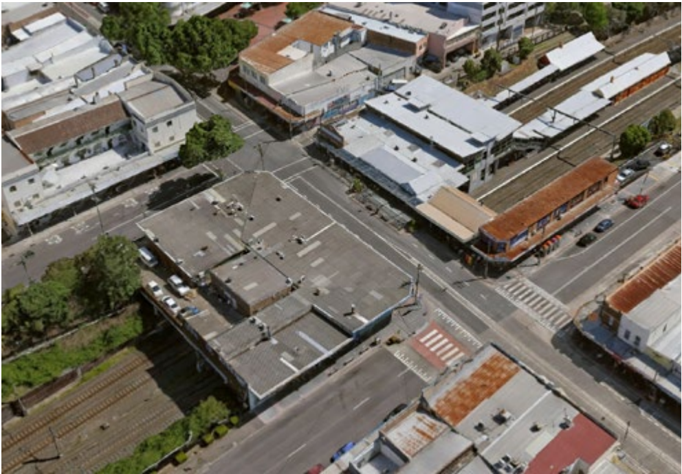
Figure 4.35 Aerial view of the existing over bridge condition at Beamish Street, Campsie
