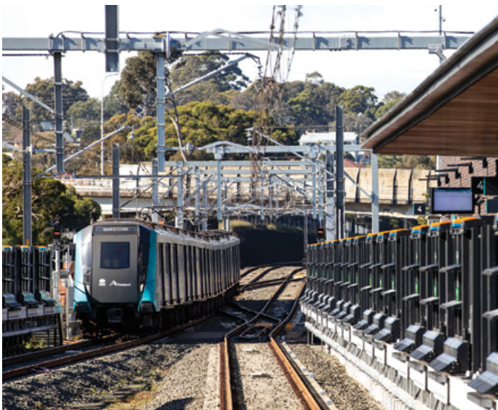
Train testing continues between Tallawong and Bankstown.
