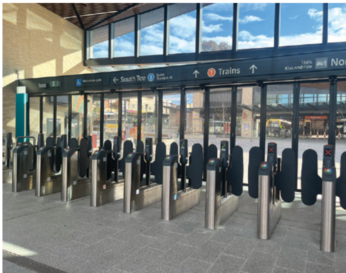
Opal gates at Bankstown Station.
