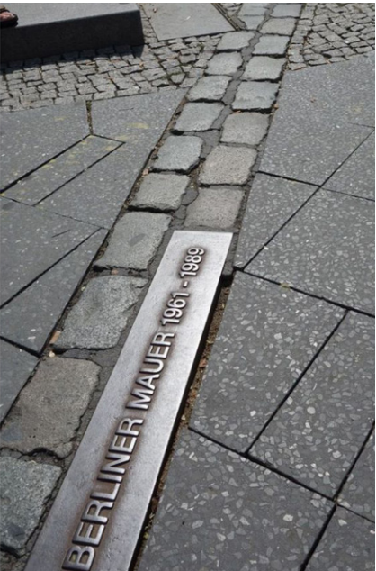
Figure 4.12 Paving inlay sample
