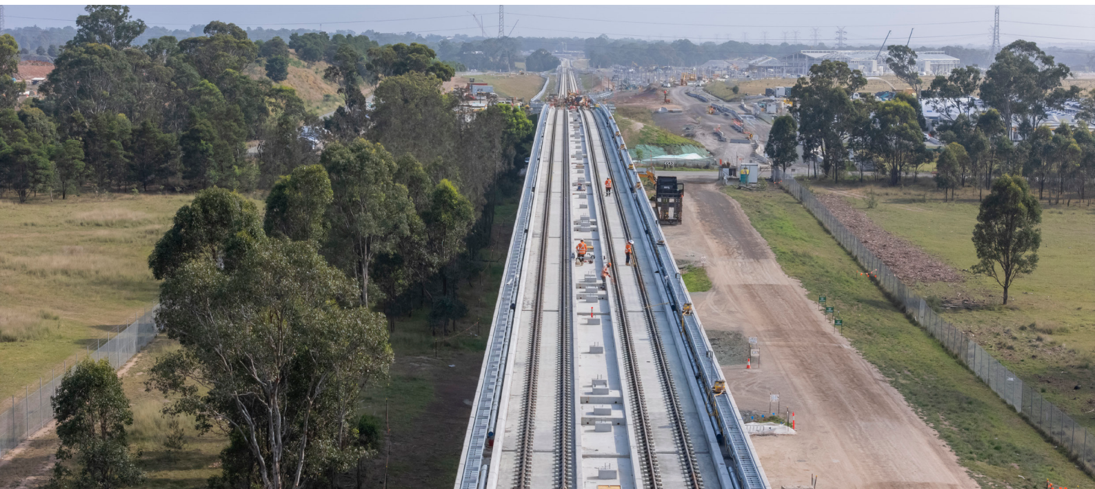
Final tracks have been laid on the Sydney Metro -Western Sydney Airport line.
