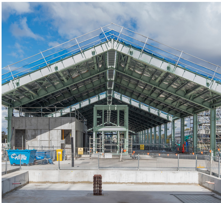
Installation of the roof canopy steel at Orchard Hills Station.
