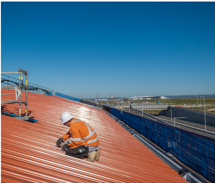
The new station roof is taking shape as sheeting works continue across the canopy and awnings.
