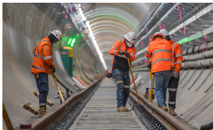
Track installation inside the Sydney Metro -Western Sydney Airport line tunnels.
