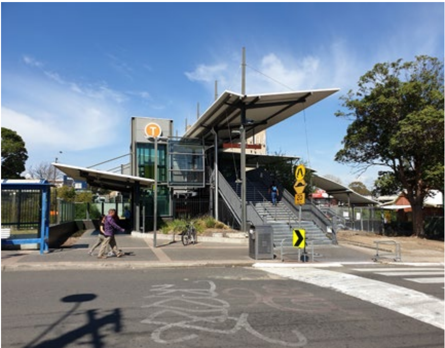
Figure 4.8 Existing station entry from Railway Parade
