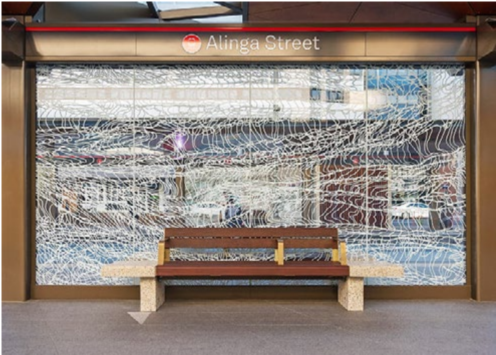
Figure 4.26 Example of glazed artwork screens at Canberra Lightrail. Art by Hannah Quinlivan
