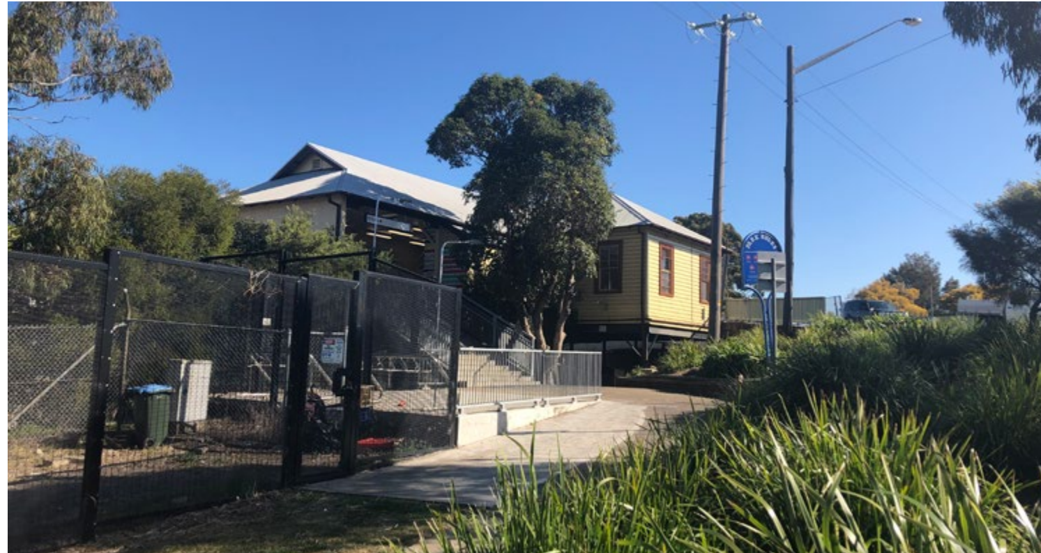
Figure 4.24 Current conditions at northern station entry
