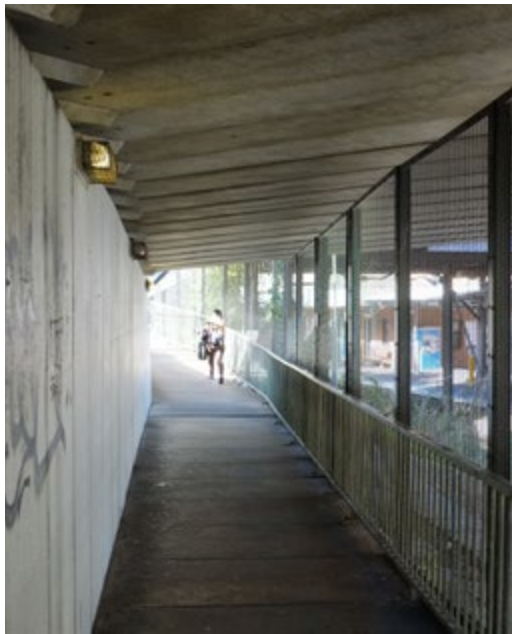
Figure 4.21 Current underpass condition
