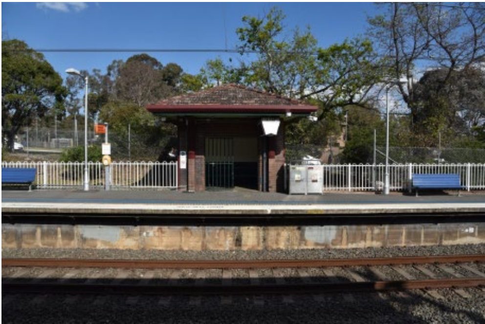
Figure 4.9 Existing waiting room current condition
