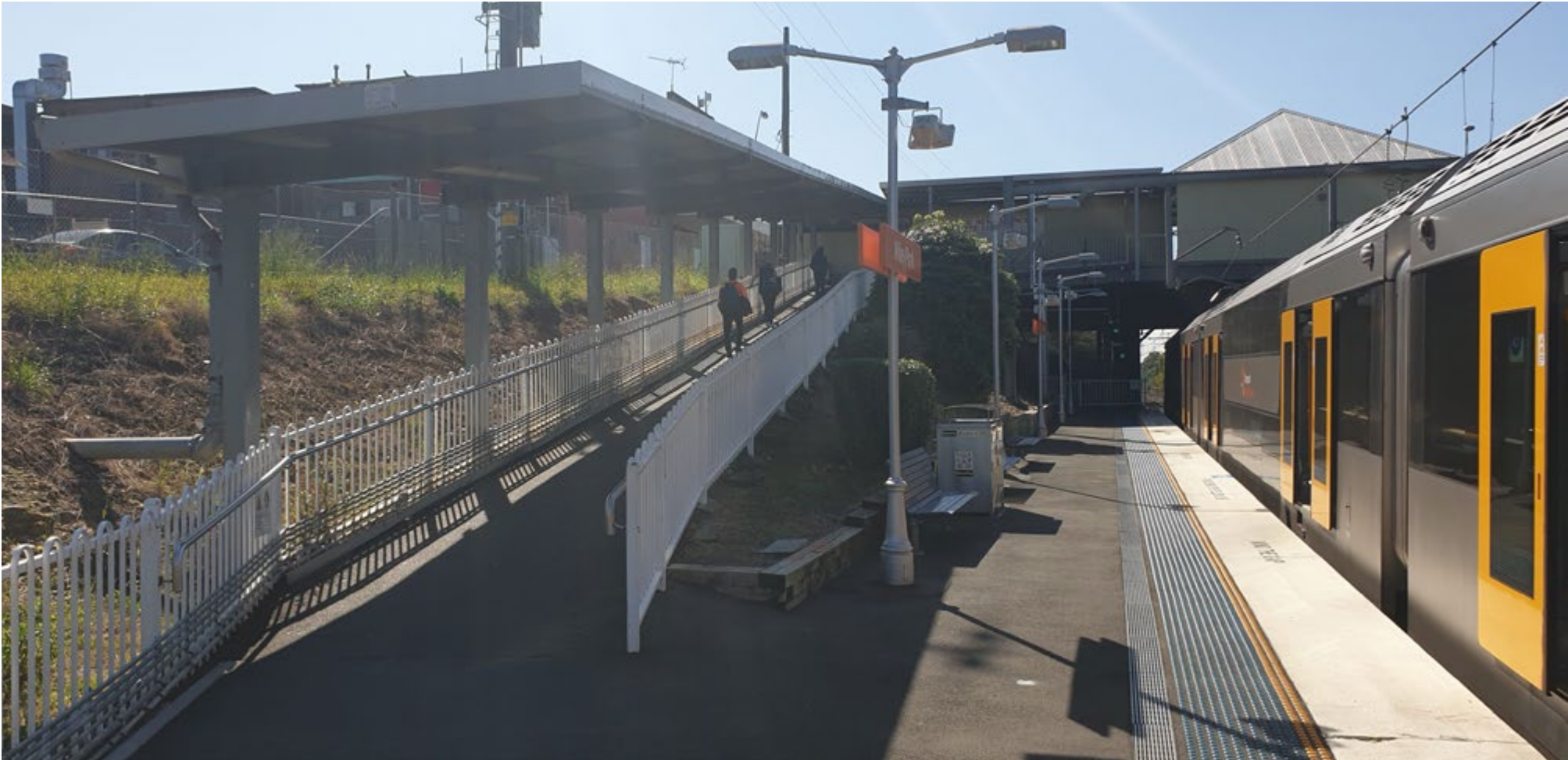
Figure 4.14 Existing ramps and canopies, platform 1
