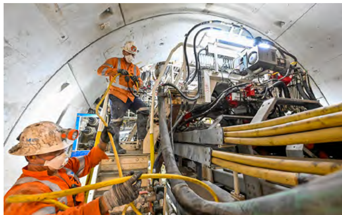
Installation of tunnel segments.
