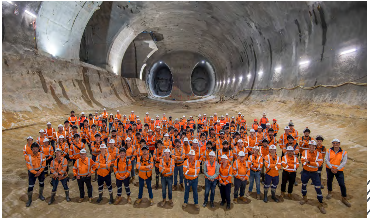
Metro West Hunter Street Station cavern.
