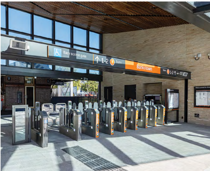
New Sydney Trains entrance with 8 new Opal gates.
