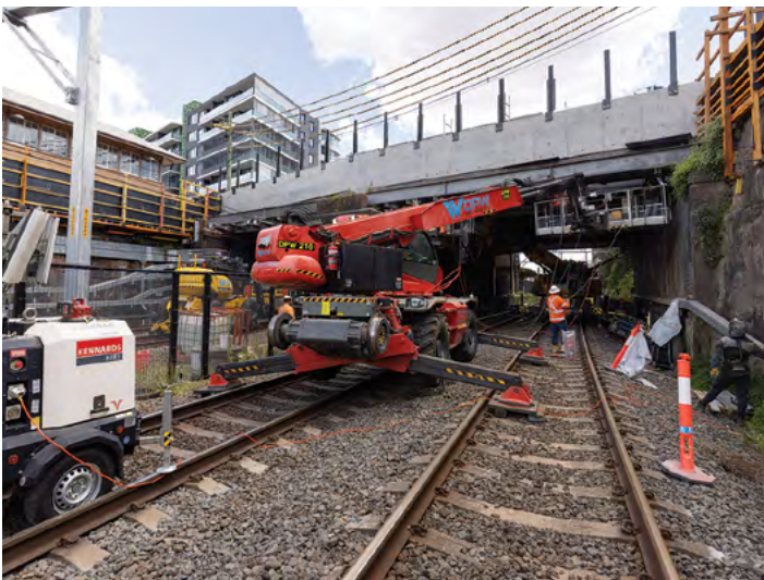
13/15 overbridges upgraded to improve safety.
