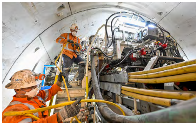
Installation of tunnel segments.
