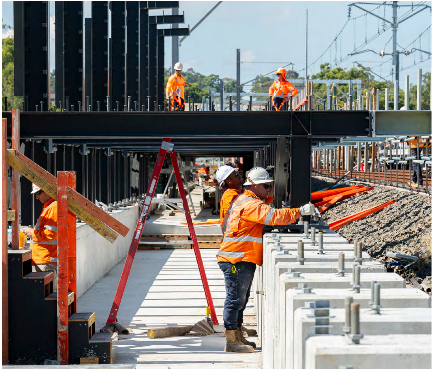
Structural steel and precast concrete panels are installed at station platform at Bankstown.
