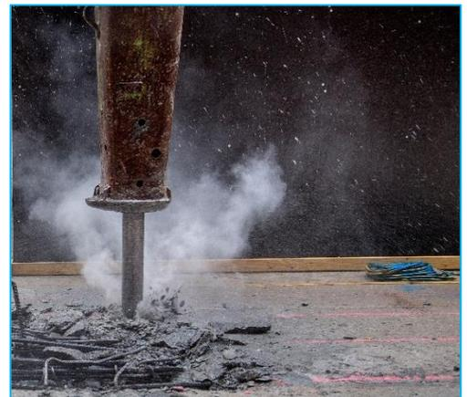
Image of excavator with hammer attachment removing concrete.
