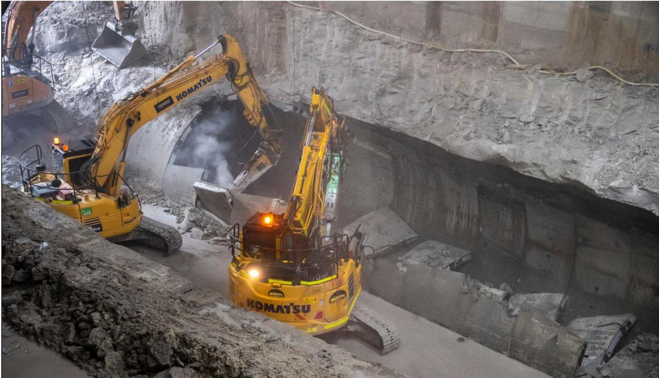
*Breaking through into the metro tunnels 27 metres under Central Station.*
