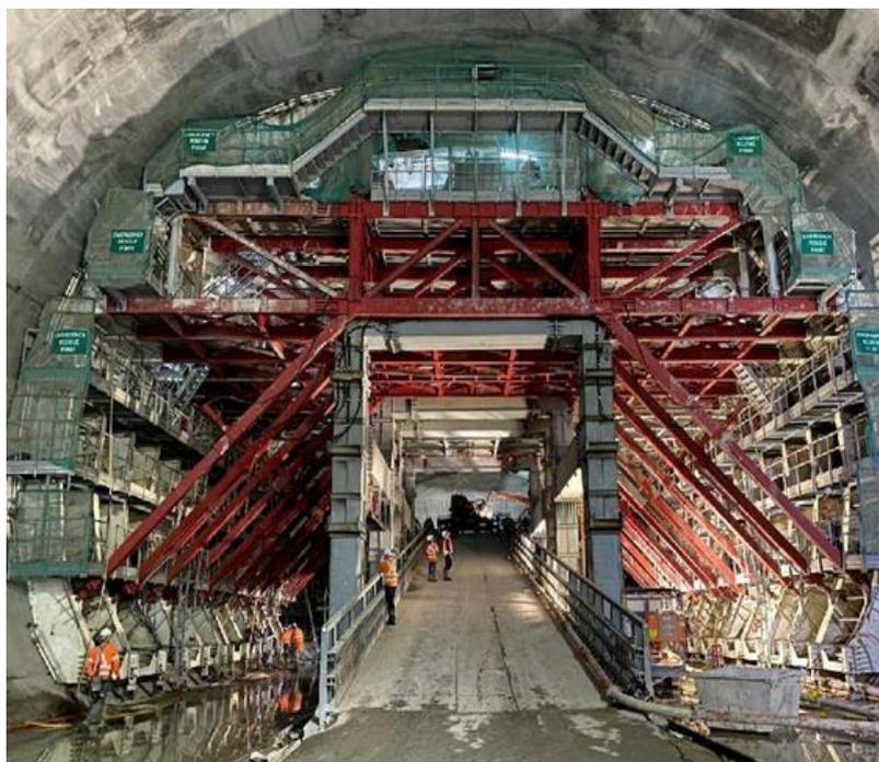
Lining the station cavern using customised steel formwork
