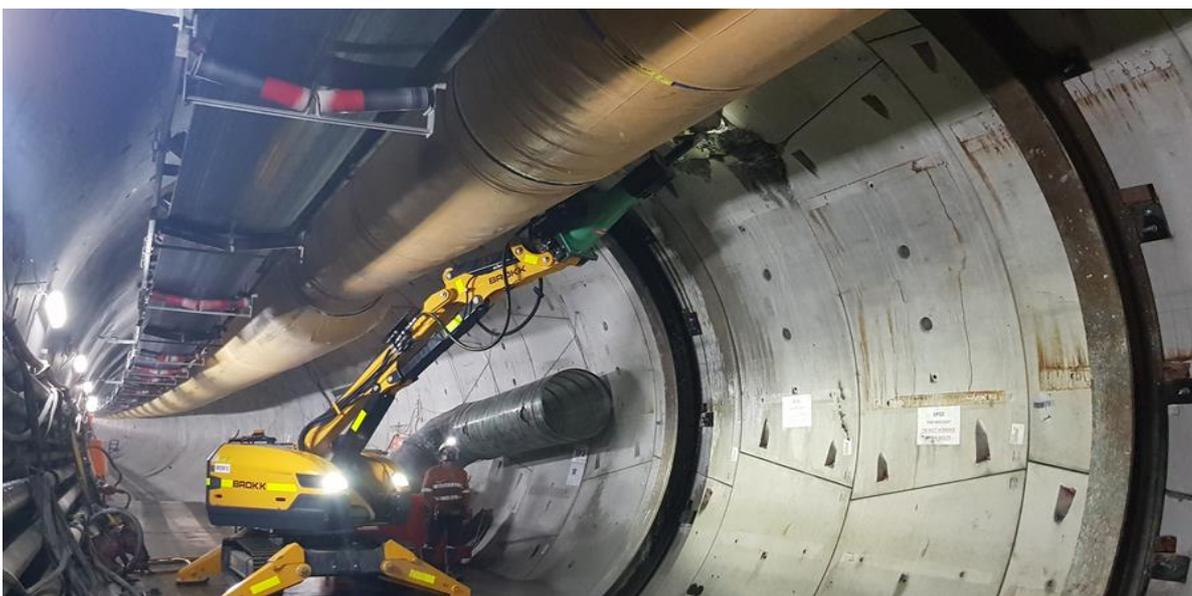
Cross passages are excavated using rock hammers like the one pictured above.
