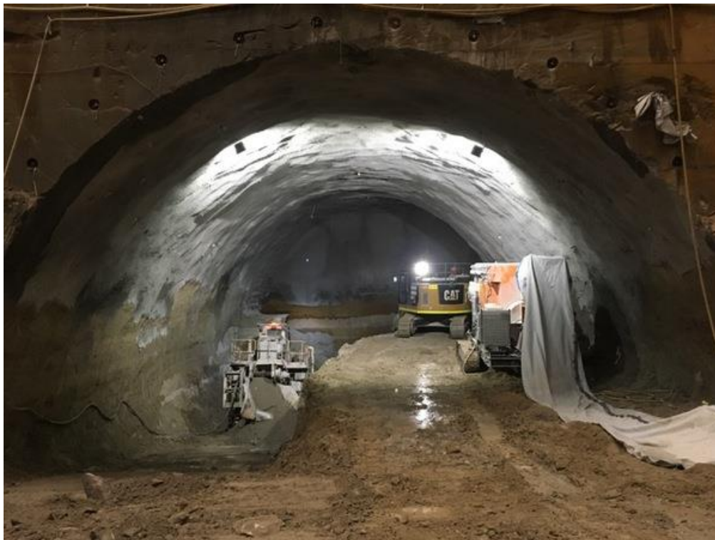
Excavation of the services tunnel under 237 Miller Street
