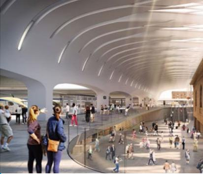
The new northern concourse will create a statement entrance to Central Station from Eddy Avenue. A new roof canopy will be installed to complement the heritage Central Electric Building and aesthetics of Central Station, and new escalators, lifts and staircases will be installed to create an open, expansive space for customers. At completion, the northern concourse will provide improved customer transport interchanges and create an entrance to the underground metro platforms.
