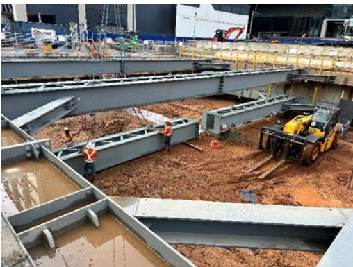
Figure 2.3: Parramatta Site – Station Box excavation
