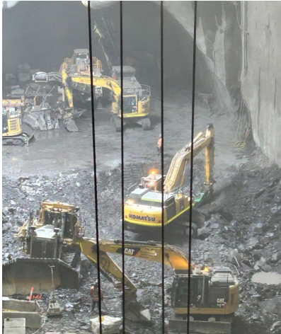
Figure 2.1: Westmead Site –Station Box excavation
