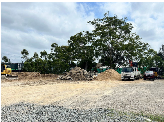
Figure 4.1: Westmead Utility Works – Silverwater Compound waste and sand stockpiles
