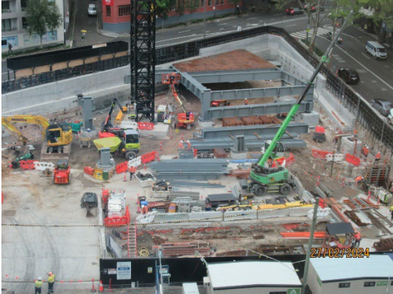
Figure 3.1 Pyrmont East: Ongoing installation of the steel platform.
