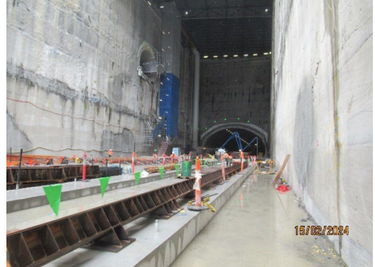
Figure 1 4 TBM traverse plinths and modules in place (Burwood North).
