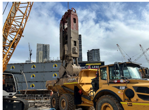
Figure 2.4: Parramatta site – D-Wall grab unloading spoil
