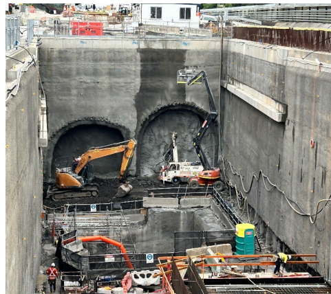
Figure 2.6: Clyde Dive site – Dive portals with water sump
