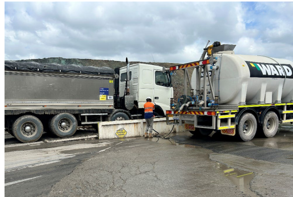
Figure 2.14: Clyde MSF Site – Wheel wash with hose cleaning tyres
