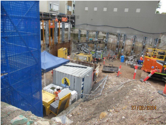
Figure 3.3 Pyrmont West: Anchor installation. Wall supports in place.
