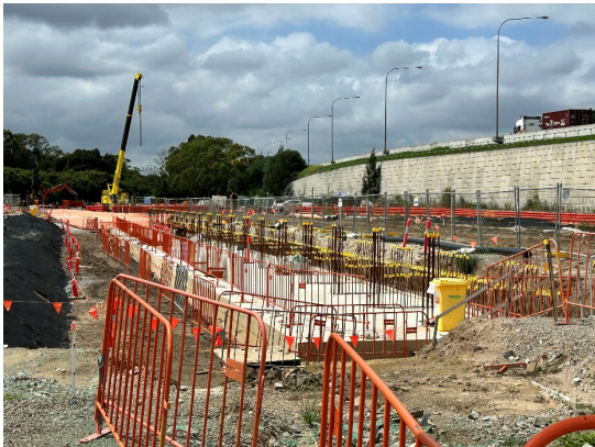
Figure 2.13: Clyde MSF Site – Utilities retaining wall construction
