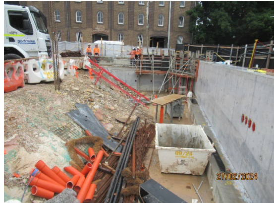
Figure 3.4 Pyrmont West: Construction of retaining wall along Paternoster Row and Pyrmont Bridge Road.
