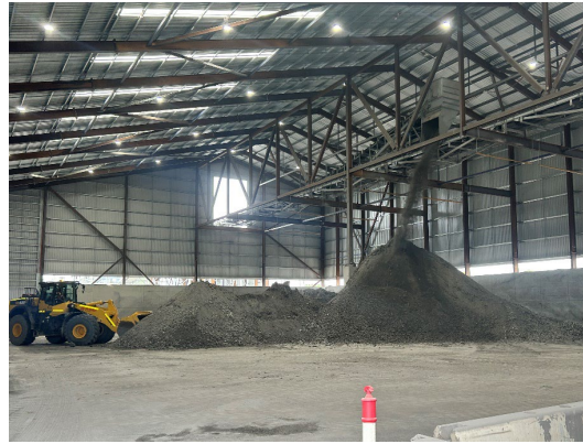
Figure 2.10: Rosehill Site – TBM Spoil shed
