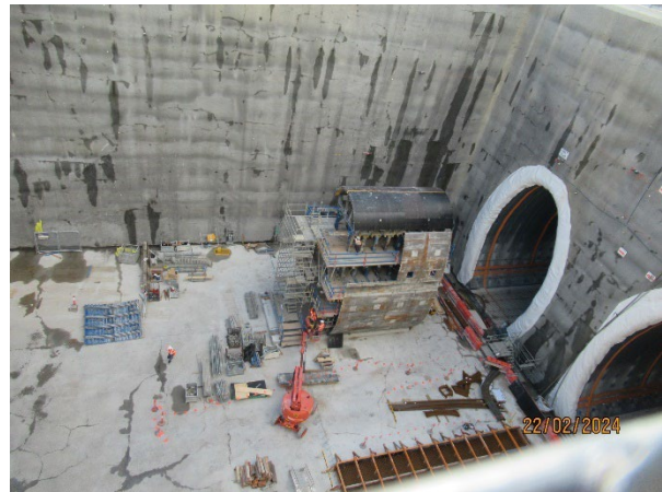
Figure 1.8 Assembly of formwork structure for lining of the nozzles (SOP).
