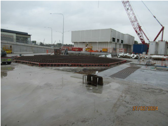
Figure 3.7 The Bays: Ongoing construction of the Slurry Treatment Plant
