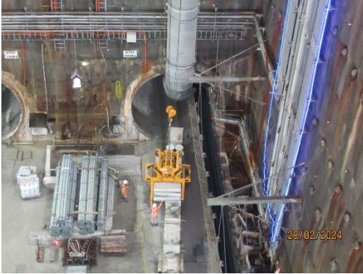
Figure 1 1 The western end of the station box (The Bays).
