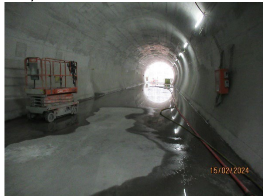
Figure 1 6 Pedestrian Tunnel (Burwood North).
