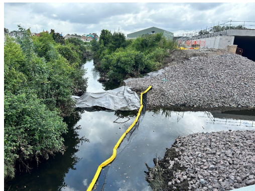
Figure 2.12 – Clyde MSF Site – A'Becketts Creek low flow construction
