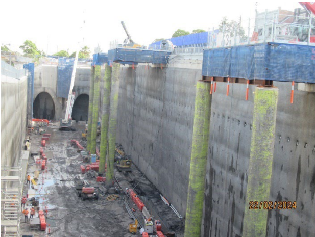
Figure 1.7 Excavation of service trenches (North Strathfield)
