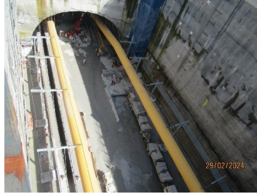
Figure 1 2 TBMs not visible in the Western Shaft (Five Dock).
