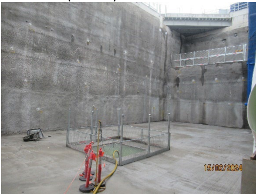
Figure 1 5 South Shaft completed (Burwood North).
