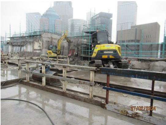
Figure 3.5 Hunter St West: Demolition of the core of building on Level 19
