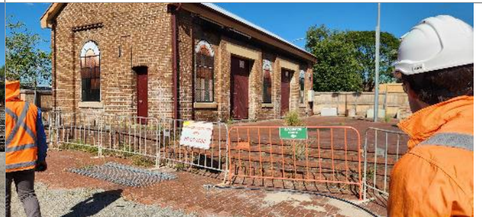
Photo 6 – St Marys historic goods shed
