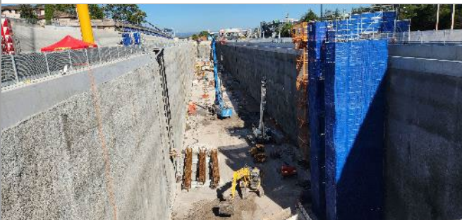
Photo 7 – St Marys station box excavation site
