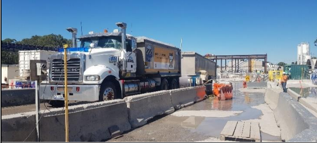
Orchard Hills – Automated wheel wash.
