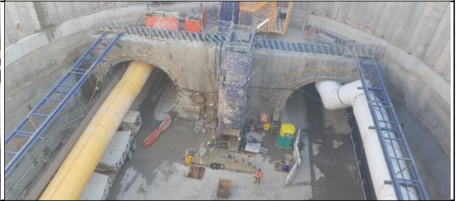
Claremont Meadows shaft view north – Tunnel segment loading into tunnel.
