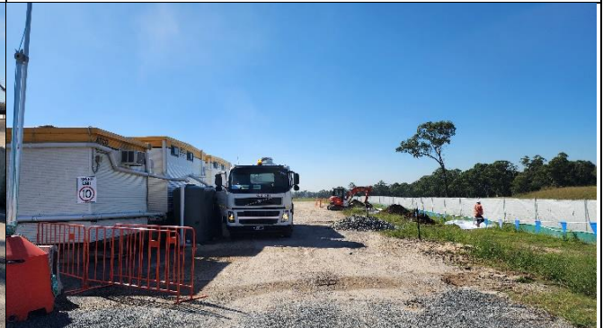
SMF – Installation of water discharge to swale from the office compound.
