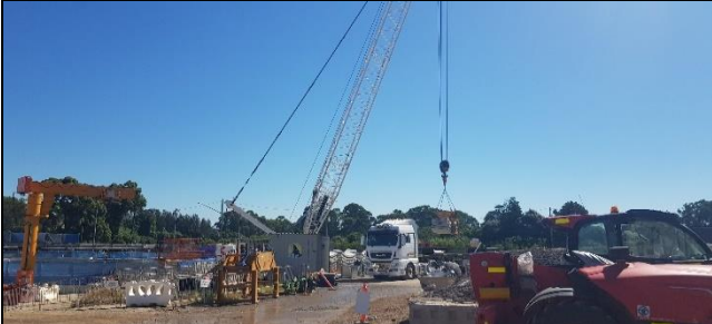
Claremont Meadows shaft view north – Tunnel segment delivery from Orchard Hills.
