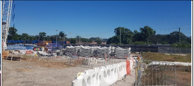
Claremont Meadows north west – Tunnel segment storage.
