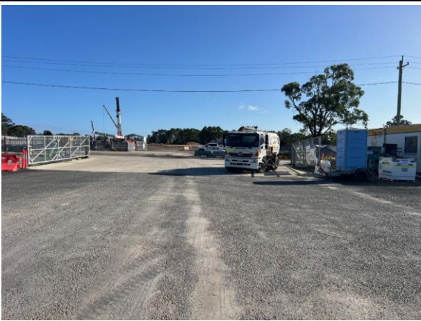
Lansdowne Rd – Following ER inspection on 07/03/24 a street sweeper is stationed full time at the SCAW Lansdowne Rd exit
