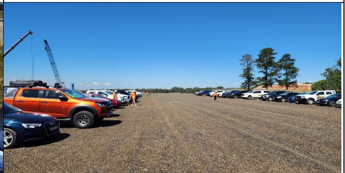
AEC – It was noted that the light vehicle road and car park had been constructed
