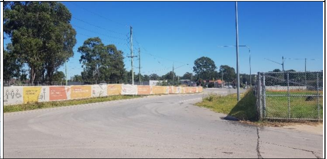
Claremont Meadows – Negligible tracking noted from southern site access onto Gipps Road.
