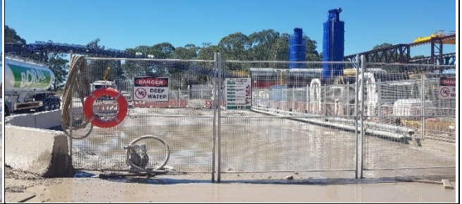
Orchard Hills south – CPBG to empty water holding sumps to allow for unpredictably intense rain events.
