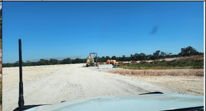
SMF – Water truck refilling from sump
