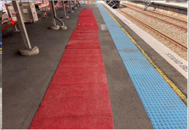
Platform - A red carpet has been provided to identify the walkways and reduce the amount of mud tracked by foot traffic.
