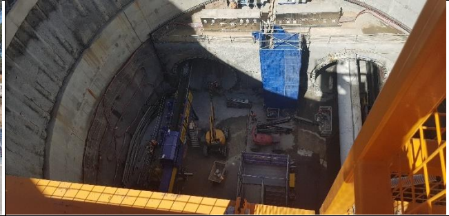
Bringelly facility - Installation of tunnel ventilation and spoil conveyor boosters.
