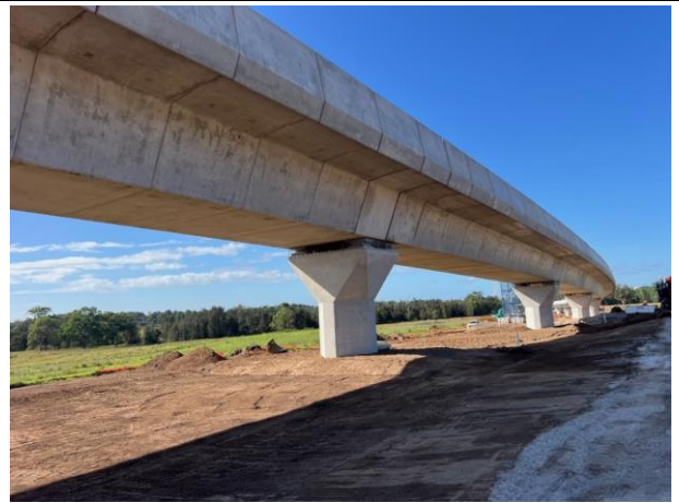
Luddenham South - The viaduct works are complete at Luddenham South
