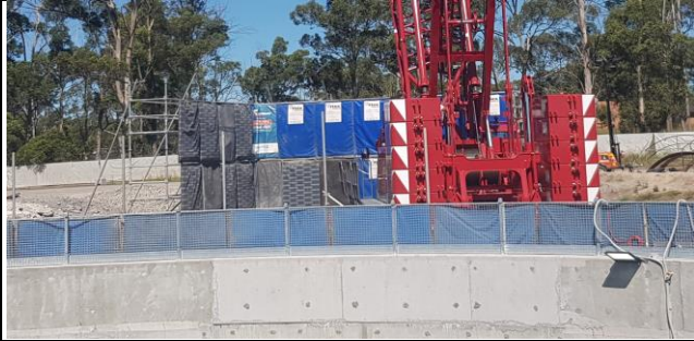
Bringelly Facility view southwest – CPBG to orient absorptive surface of noise blankets towards works.
