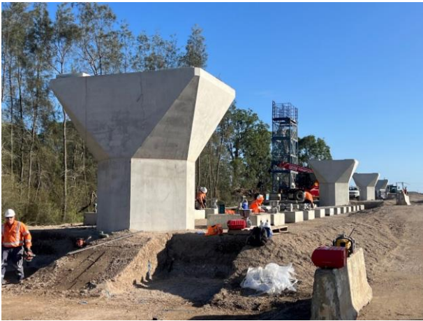
Defence - Structures works are ongoing in the Defence site
