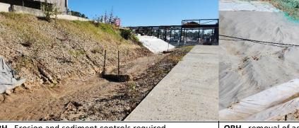
**ORH** –Erosion and sediment controls required maintenance. A 30m section of the embankment was pending the application of soil binder. **ORH** –removal of accumulated sediment was required on the SBT boundary. Soil binder had been applied to the embankment.
