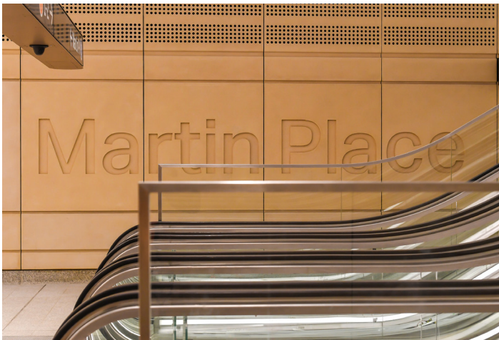
Martin Place signage embossed in glass reinforced concrete (GRC) located in the arrivals hall on the platform.
