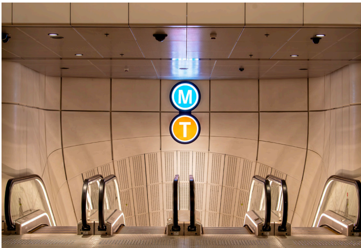
View of the incline escalators transporting passengers from the southern concourse to station platforms.
