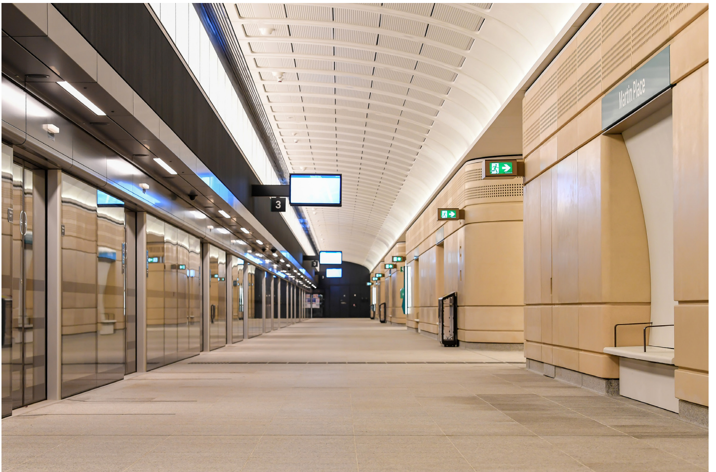
The eastern platform runs 25 metres directly below Elizabeth Street and is 210 metres long.
