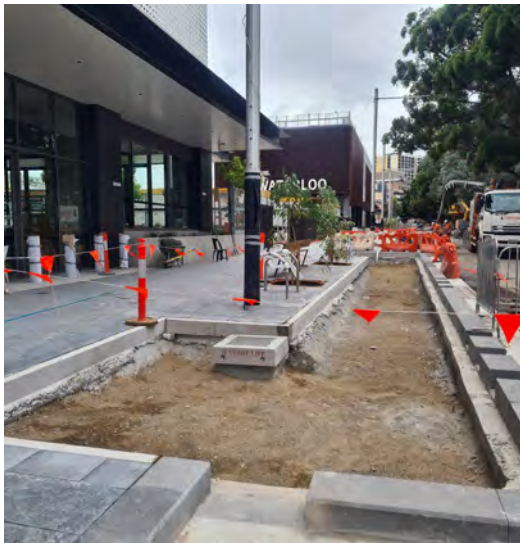
Cope St: Landscaping and planting work; kerbing, paving and rain garden construction on Cope St continuing.
