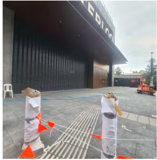
WL ISD: Paving installed at Station entrance - Raglan St.
