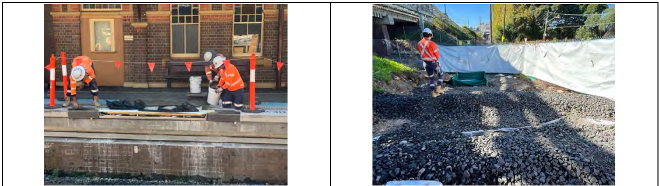
Installation of MGFs on platforms, Marrickville Station.
