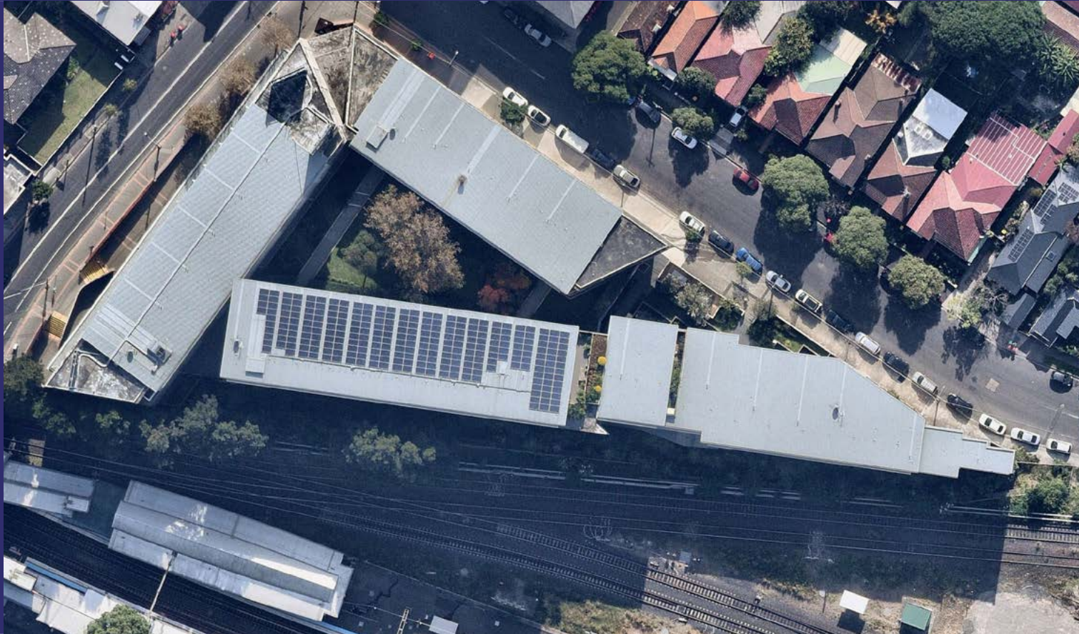
Renewable energy: Solar panels at Marrickville Station.
