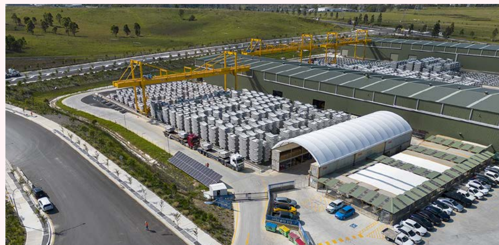
Manufacturing segments: Eastern Creek precast facility where over 60,000 segments will be manufactured.
