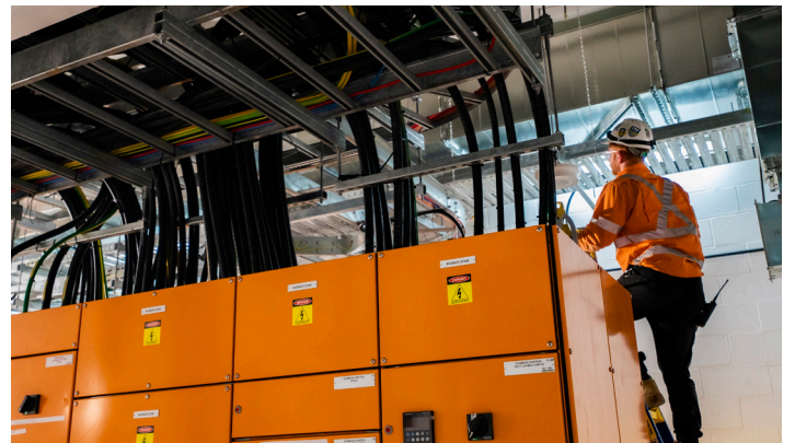
Workers are testing electrical cables and equipment at the trains facility.
