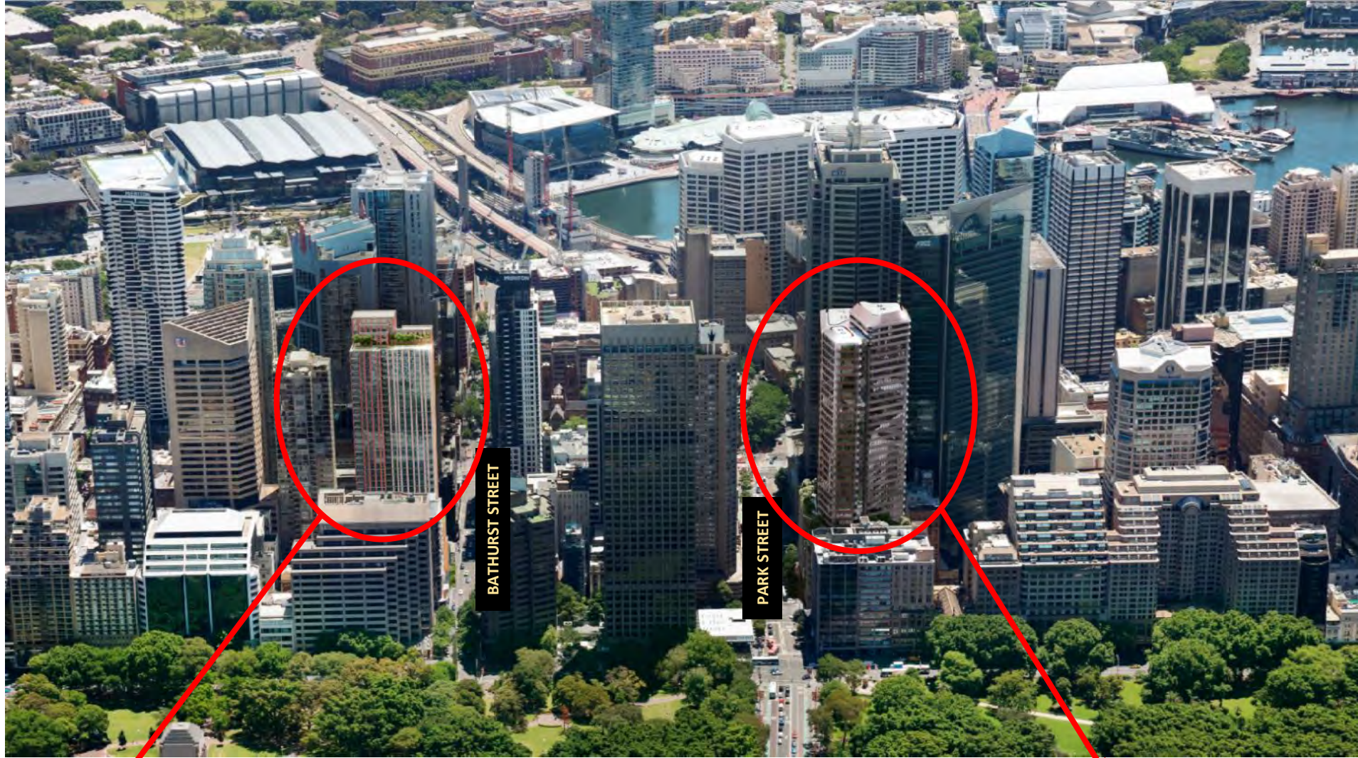
South Station and Tower (OSD)
