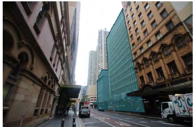
Picture 5 View prior to building demolition (2016)
