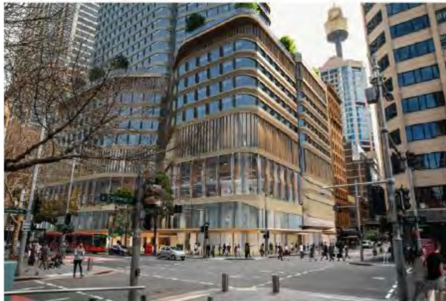
Figure 38 – Artist's impression of north station podium viewed from south west (source: Arterra Interactive)
