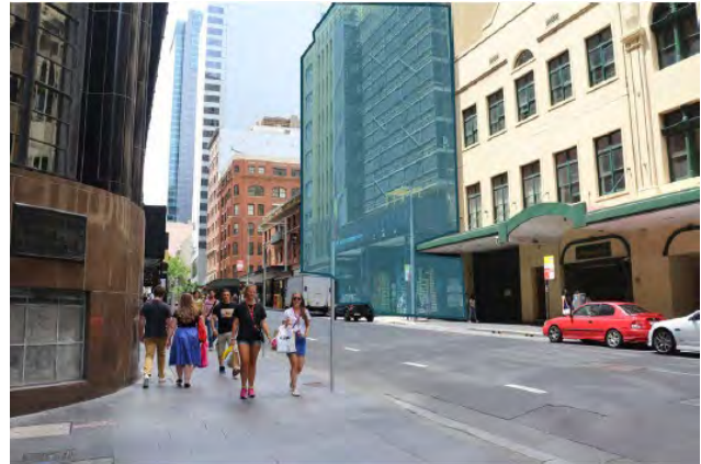
Picture 26 View prior to building demolition (2016)
