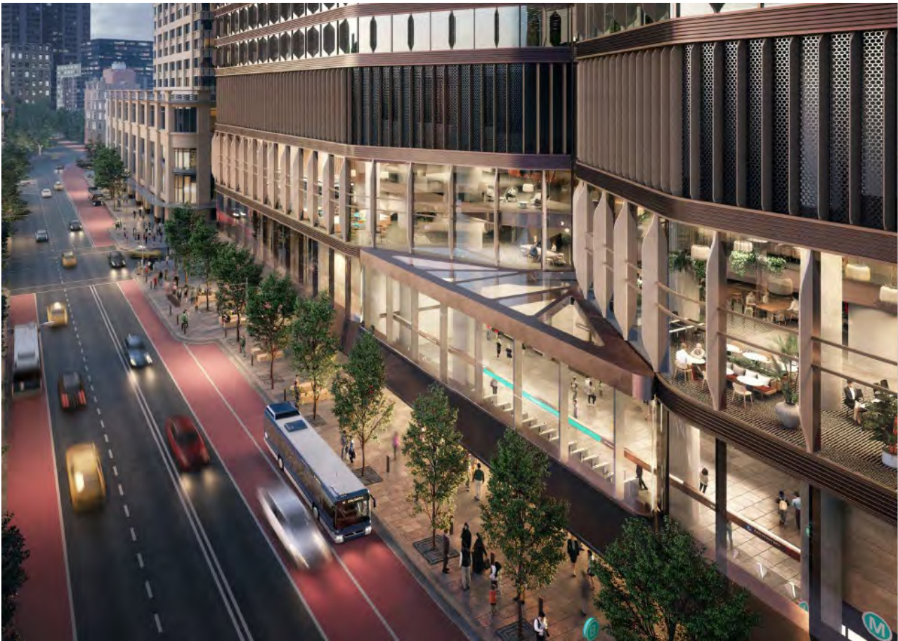
Figure 1 Pitt Street north station entrance fronting Park Street
