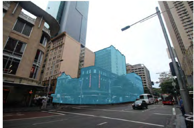
Picture 14 View prior to building demolition (2016)
