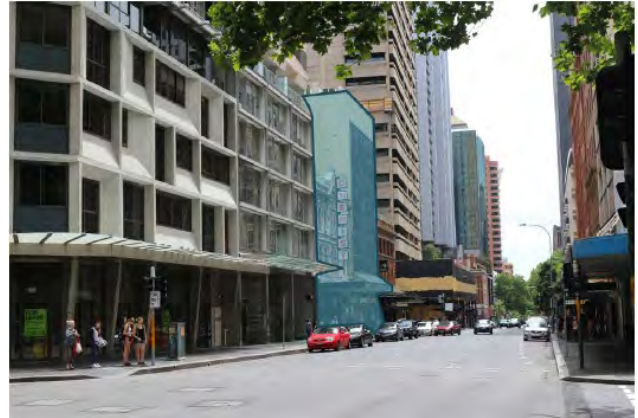
Picture 20 View prior to building demolition (2016)
