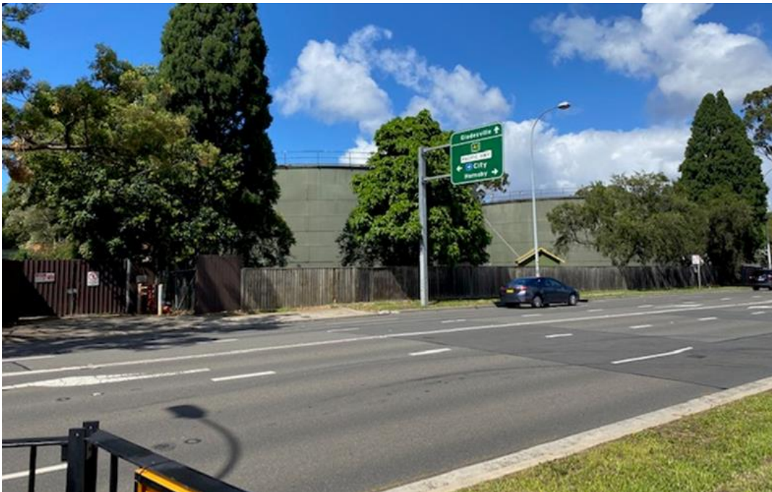
Figure 19 – View SW from Mowbray House to Chatswood Reservoirs.
