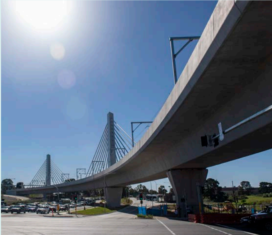
Windsor Road Bridge in Rouse Hill, part of the Metro North West Line.
