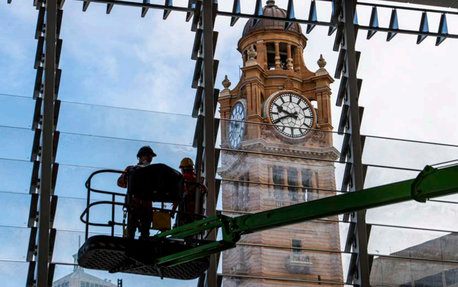
Sydney Metro construction at Central Station's northern concourse.
