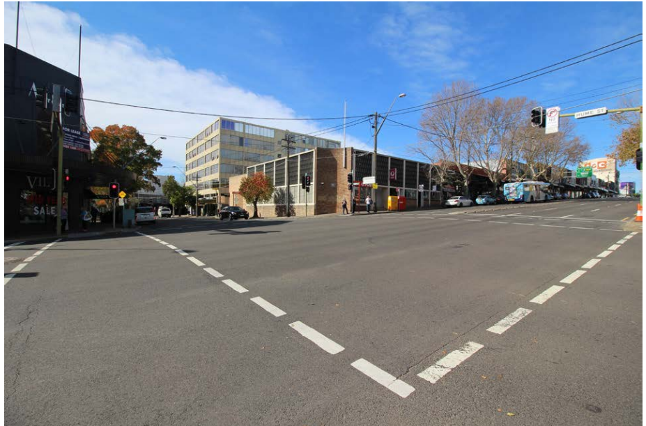
05 Pre-construction view east from corner of the Pacific Highway and Hume Street
