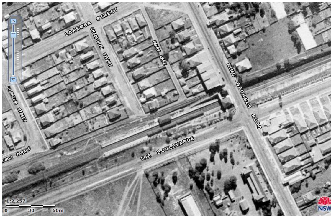
Figure 87. Wiley Park Station in 1943. Source: Lands and Property Information, SIX Maps.
