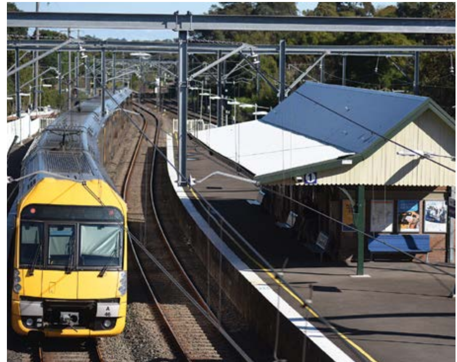
All heritage buildings along the Bankstown Line will be retained
