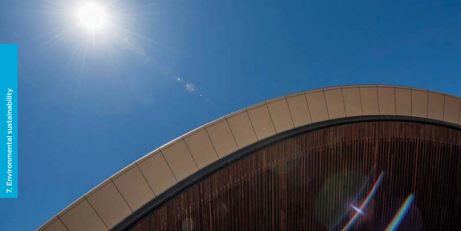
Forest Stewardship Council timber installed at Tallawong Road Sydney Metro Northwest Station.
