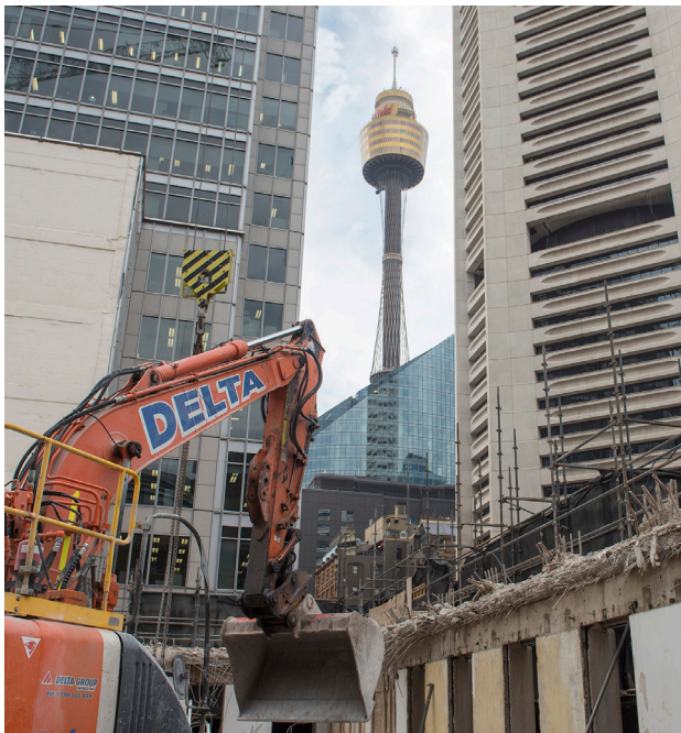
Demolition and excavation at Martin Place.
