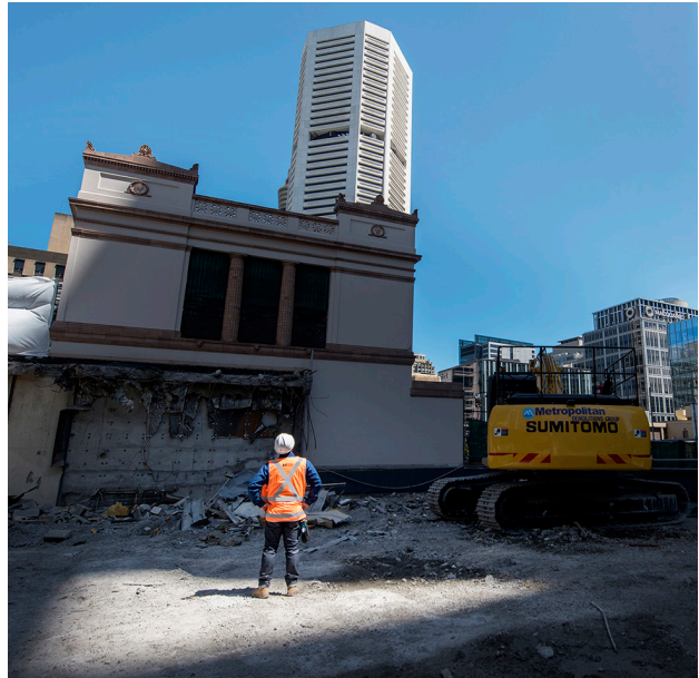
Demolition at Martin Place North, Hunter Street.
