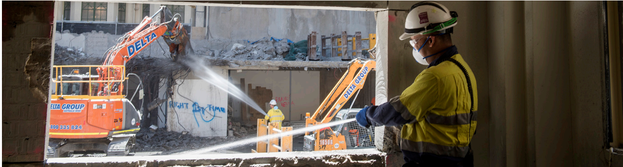
Demolition at Pitt Street North.
