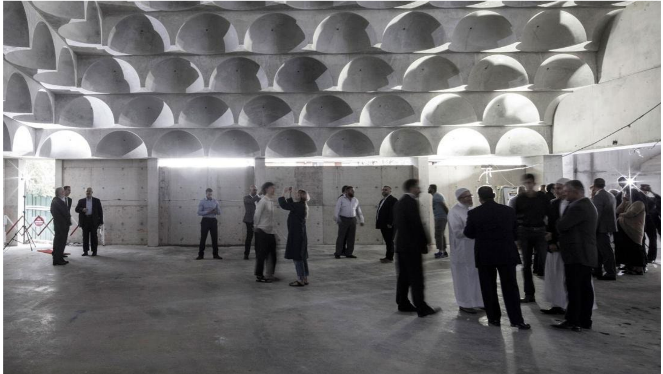
Figure 3.6 Punchbowl Mosque. Image credit Brett Boardman
