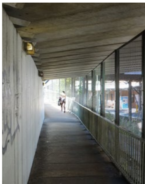
Figure 4.21 Current underpass condition
