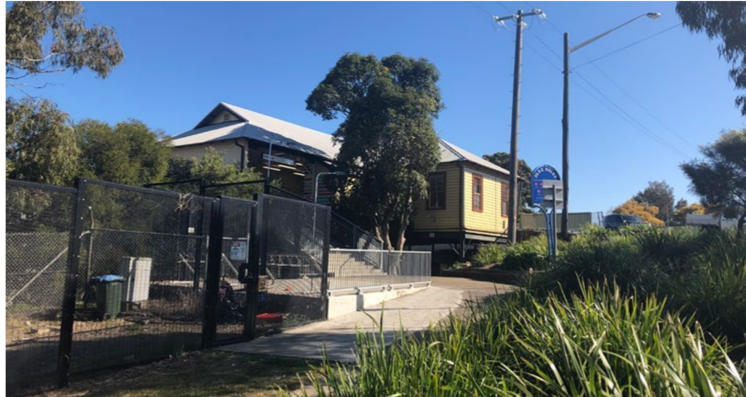
Figure 4.24 Current conditions at northern station entry
