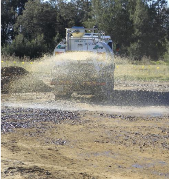
Photo courtesy of Roads and Maritime Services.
